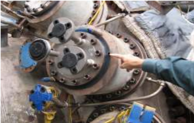
Figure 2 – Location on the Top Hat where the Transducer is Inserted
